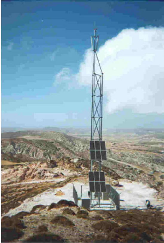
Figure 2: Installed PV-based T/C station in Greece
