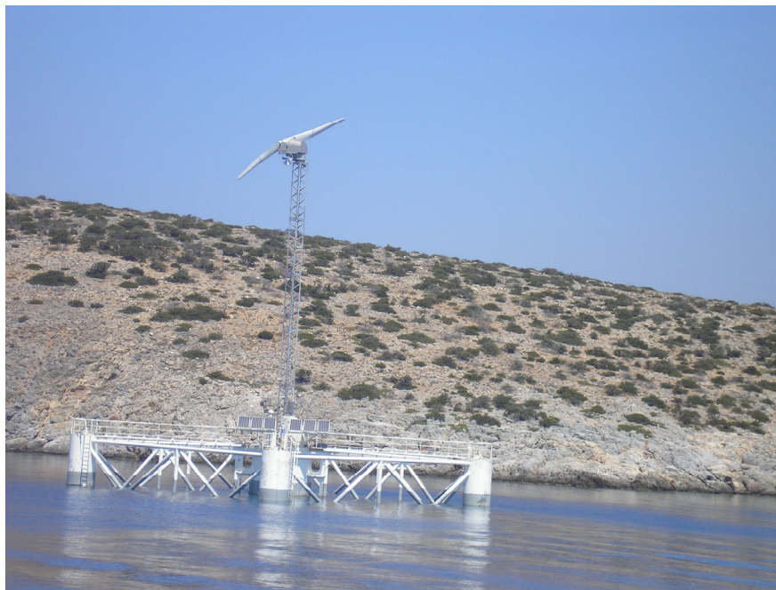
Figure 4: Floating Desalination Unit in Heraklia's harbour
